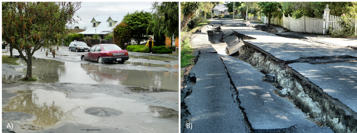
Figure 2-1. Water-saturated sand can turn to quicksand during strong shaking, forming sand boils, ponding, and sunken roads. In these examples, (A) extensive liquefaction occurred along River Road in Christchurch, New Zealand following the February 2011 earthquake, while (B) effects from lateral spreading along numerous Christchurch roads constructed next to waterways resulted in major failures to road infrastructure as roads slumped toward river channels. During a Cascadia subduction zone event, such processes could compromise tsunami evacuation routes as well as the time and speed to safety in areas prone to liquefaction. (Photo credits: Martin Luff, licensed under CC BY-SA 2.0)
